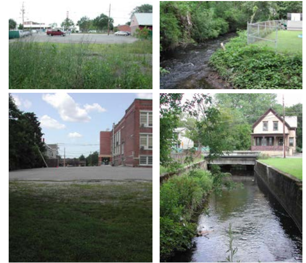
Flood control remediation issues: unmediated runoff from parking lots; eroded banks; restrictive channeling; inadequate bridge apertures
