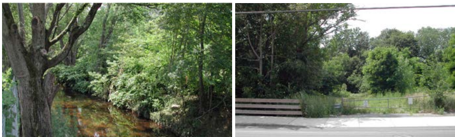
Salisbury Brook runs into Calhoun Green from open banks into channelized stream (under Warren Avenue) contributing to the flooding in this area.
