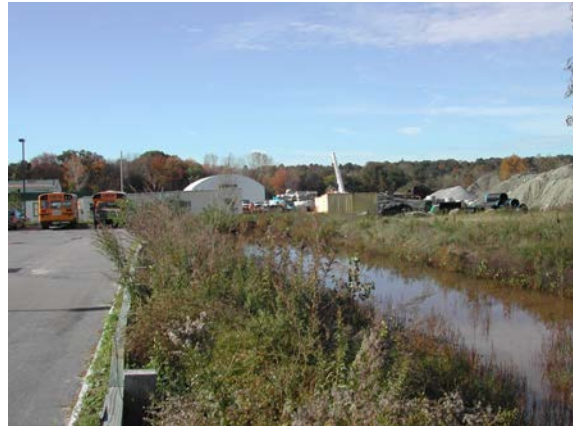
The detention basin adjacent to the school car park and the neighboring sand quarry does not have a sufficient buffer zone to adequately filter noxious effluent. Additional planting and a curb at the edge of the parking area will alleviate some of the ill effects of these adjacencies.
