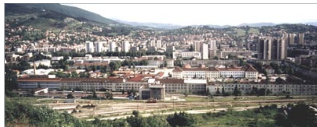
Military Barracks, View from North
