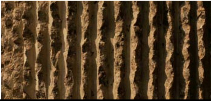
Above: Lindemann Center (Paul Rudolph, 1970). Coarse-aggregate concrete was poured into corrugated form liners and bush-hammered.
