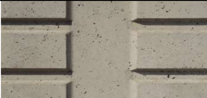
Below: Viaduct piers, new Central Artery (Wallace Floyd Associates with Stull and Lee, 1992). Rustication detail creates a sense of scale.
