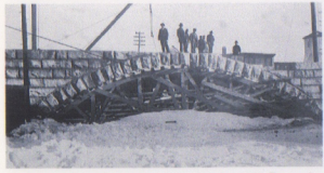
The Crescent Street Arch under construction, circa 1895. The wooden centering supporting the voussoirs (the radial stones forming the arch) is still in place. At this stage of the construction the grade level remains high for ease of working. Later, the finished road grade would be some feet lower to achieve the required headroom.
