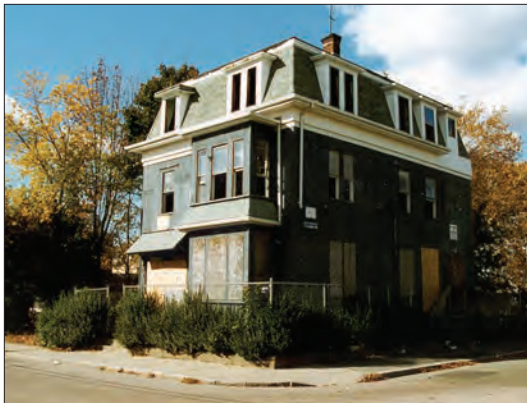
Abandoned Building - Rehabilitation versus demolition
