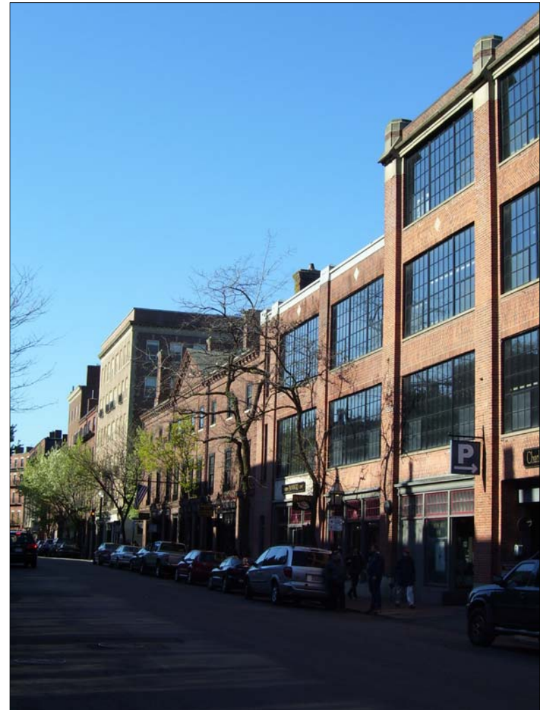
Renovated buildings may include one or more level dedicated to structured parking.
